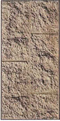
RETAINING WALL SURFACE (Concrete Split Face)
